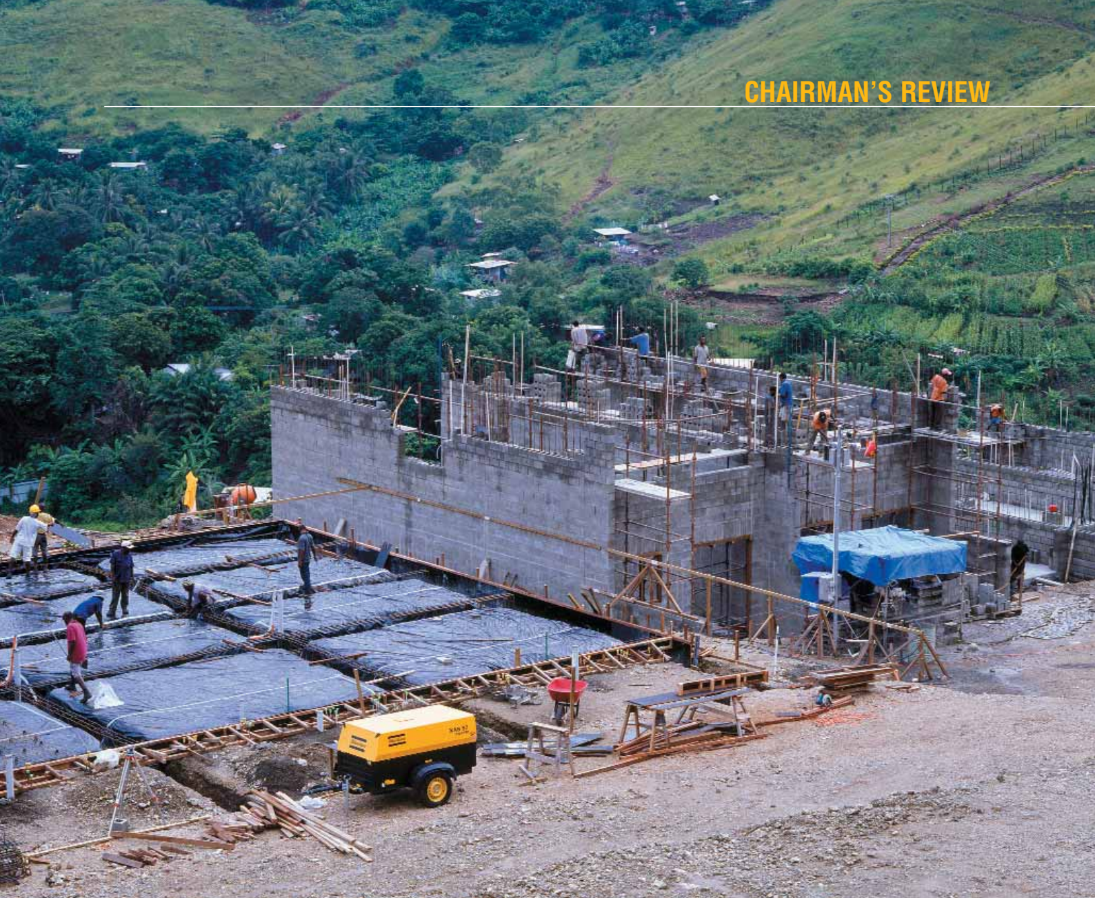
Construction of new Era Dorina Units
