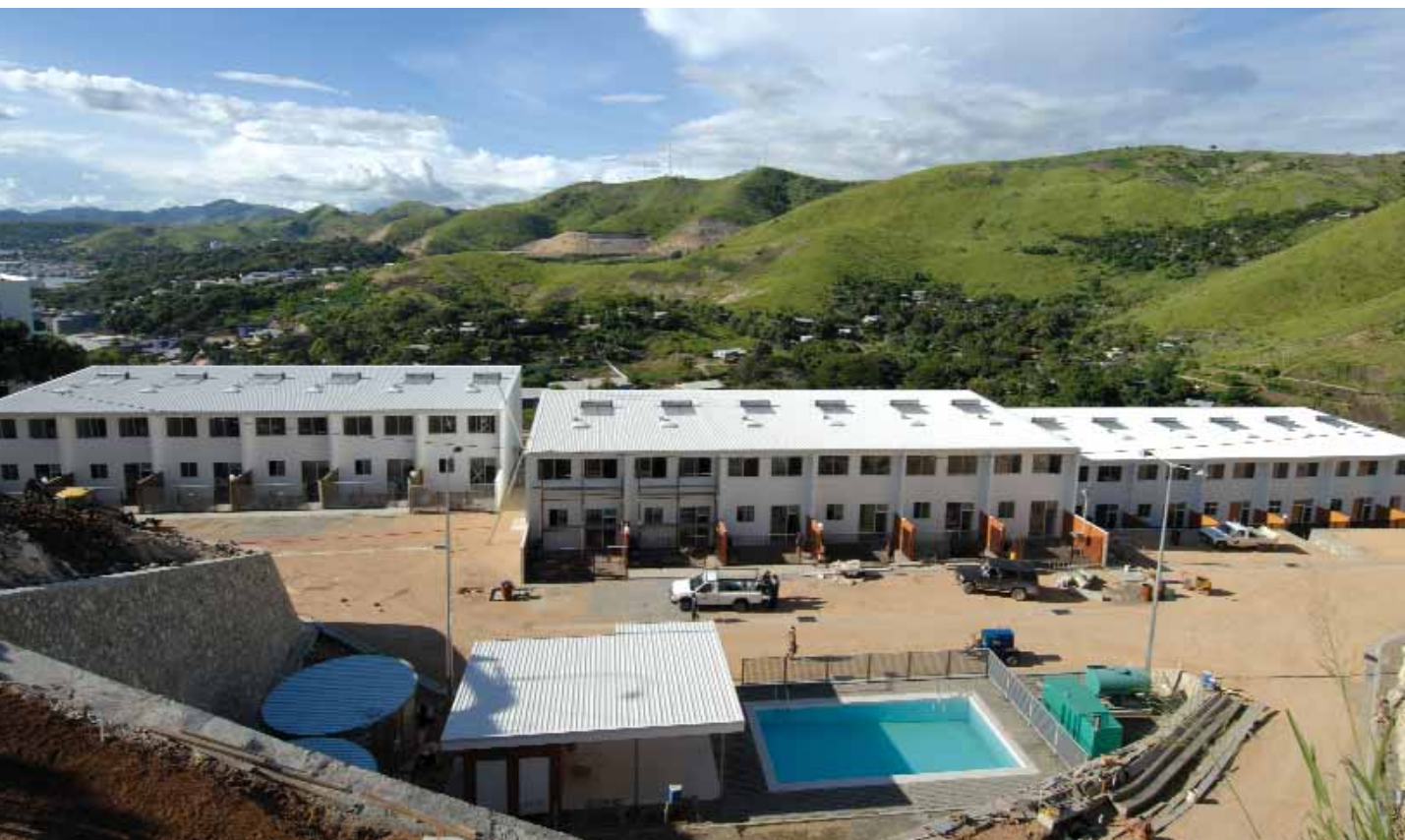
The nearly completed townhouses at Era Dorina
